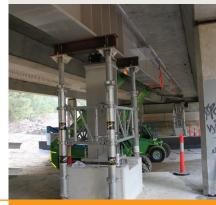
However, the use of steel girders with micro-piled foundations was the first time this methodology had been used in bridge strengthening works for an existing structure in WA. As such, it would present a number of challenges for the constructor, as no construction precedents existed.
