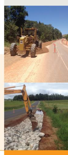
Works also included excavation and geotechnical stabilisation of an earth cutting slope adjacent to the road to remediate the effects of a recent landslide. This was achieved by drilling and grouting soil nails and rock dowels and restraining the surface using high tensile steel netting and erosion control matting. This has also significantly improved safety and driver visibility for oncoming traffic.
